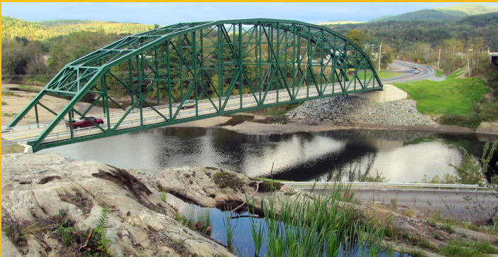
Checked House Bridge Richmond, VT
